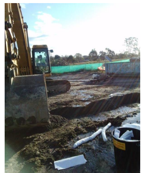
Making a dam with an excavator
